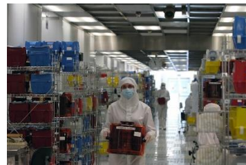
Clean room facility at LETI
